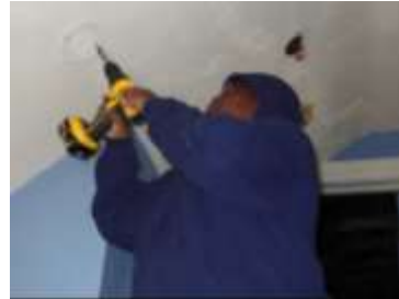
Installation of smoke detector
