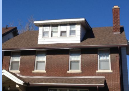
New gutters and downspouts
